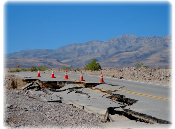
Flood damage on Highway 190
